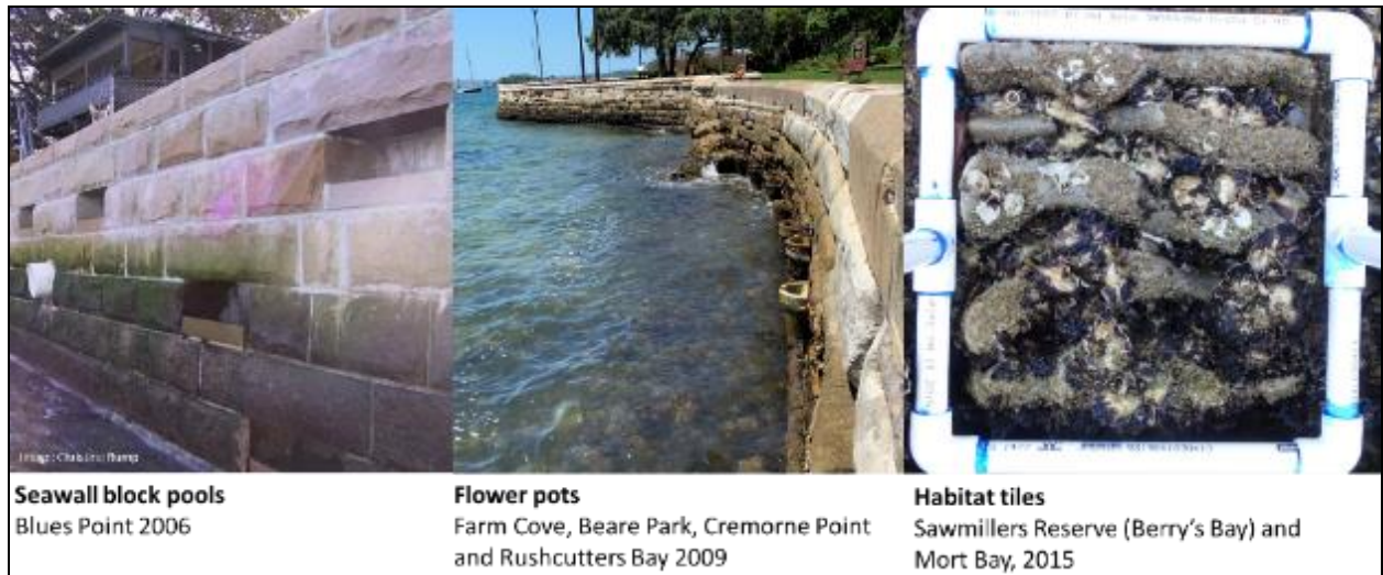
Figure 1: Evolution of early seawall “greening” initiatives in Sydney Harbour. Image credits: Christina Bump (left), Maria Vozzo (center) and Beth Strain (right).
