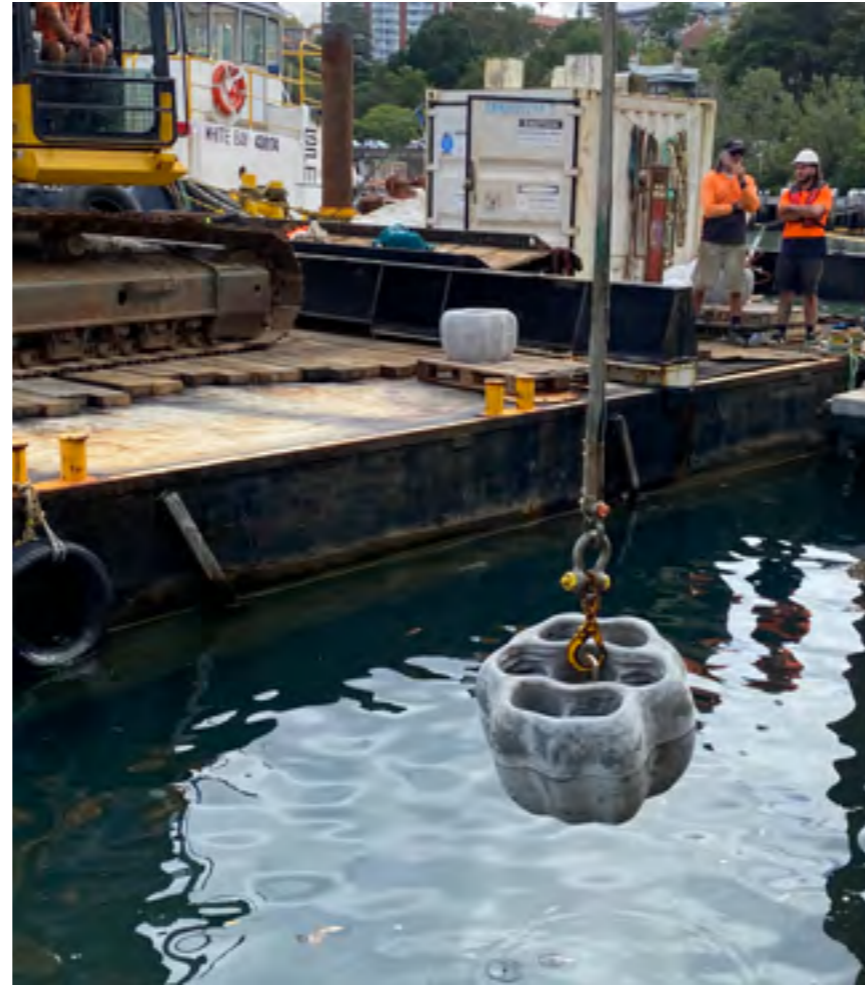
Lifters make product deployment seamless with the aid of a small crane or excavator.
