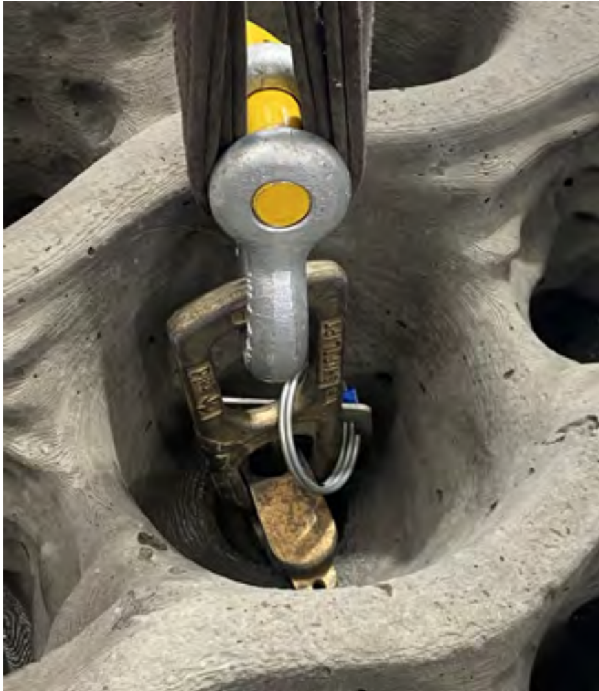
Lifters are cast within each unit and are load rated for 1300kg.
